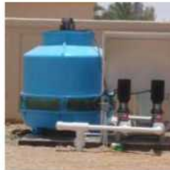
40 TR - 10 Nos RO WATER PLANT - RIYADH - KSA (2007)
