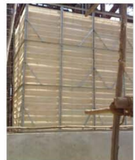
NDCT - SERIES NATURAL DRAFT COOLING TOWERS
