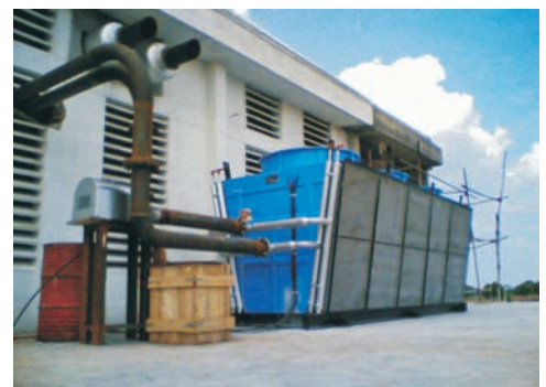
Dry-1.5Mw DG Cooling
