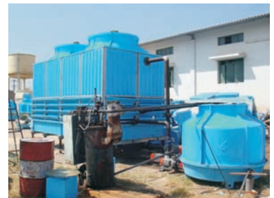
Dry-1.5Mw DG Cooling
